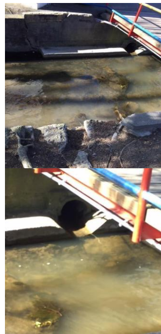
Figure 5b. Site 4 Drainage Tunnel.
