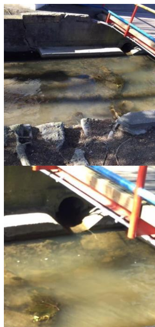
Figure 5b. Site 4 Drainage Tunnel.
